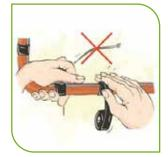
Insulate afterwards with Thermaflex tube insulation; wall thickness suited to your needs, according to the application table. Any extra length of the heating cable: fix it lengthwise at the outside of the insulation.
