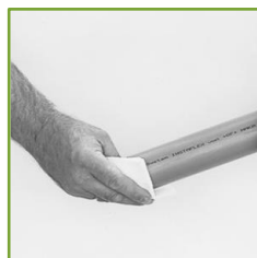
02. Clean the service pipes by using PB cleaner and tissues and make circular movements over the entire welding surface. Make sure that any printing on the service pipe is properly removed.
